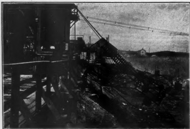
View Showing Cableway and Skip in Background with a Carriage Lowered for Repairs in Foreground
